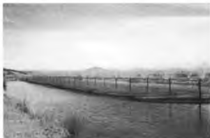
FIGURE 14-33 A spray pond.
