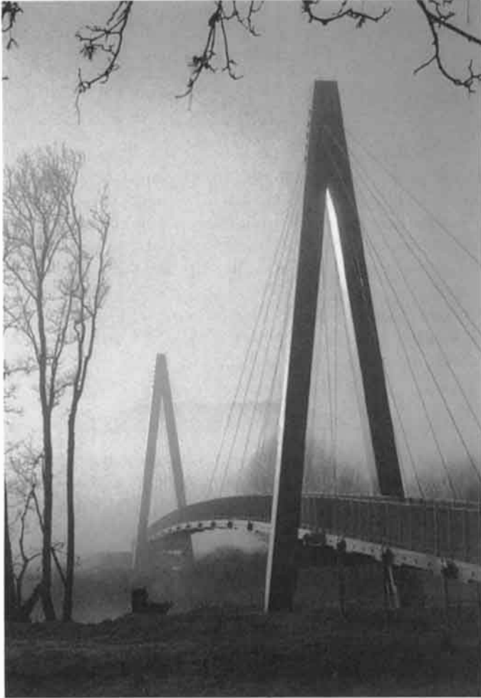
Fig. 1.20 Footbridge in Aberfeldy, Scotland, using composite decking sections. (Courtesy of Maunsell Ltd., UK.)
