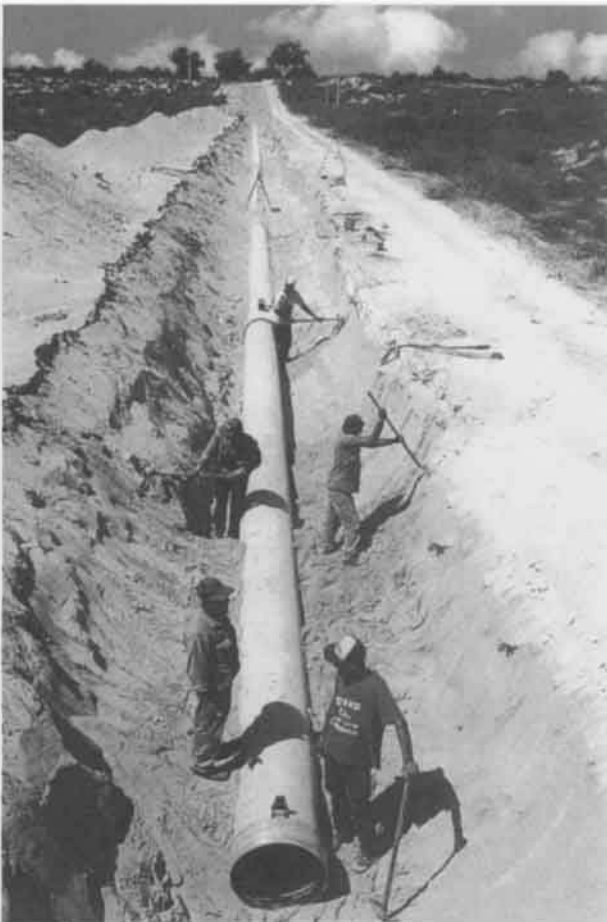
Fig. 1.19 Composite pipe used for transport of drinking water: 80 cm (32 in) diameter glass/polyester pipe. (Courtesy of FIBERTEC Fiberglass Pipe Industry, Israel.)
